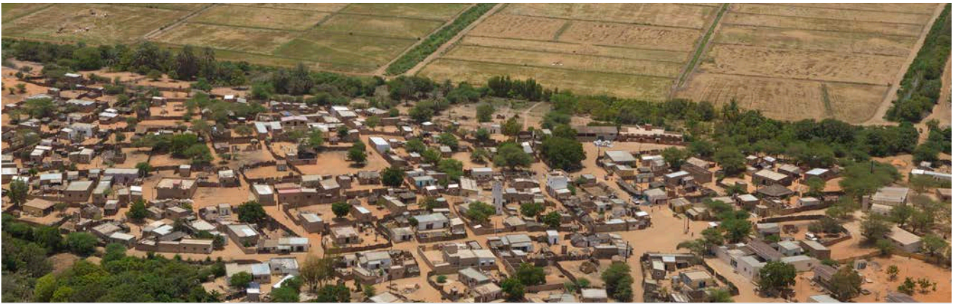
Communities and farmlands in the Senegal River Delta benefited from MCC's irrigation infrastructure rehabilitation and water resource management project. Credit: MCC
