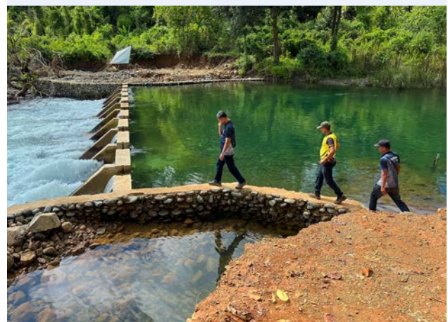
USAID Philippines supported the Palawan government to develop a climate-resilient water intake structure to supply water. Credit: USAID
