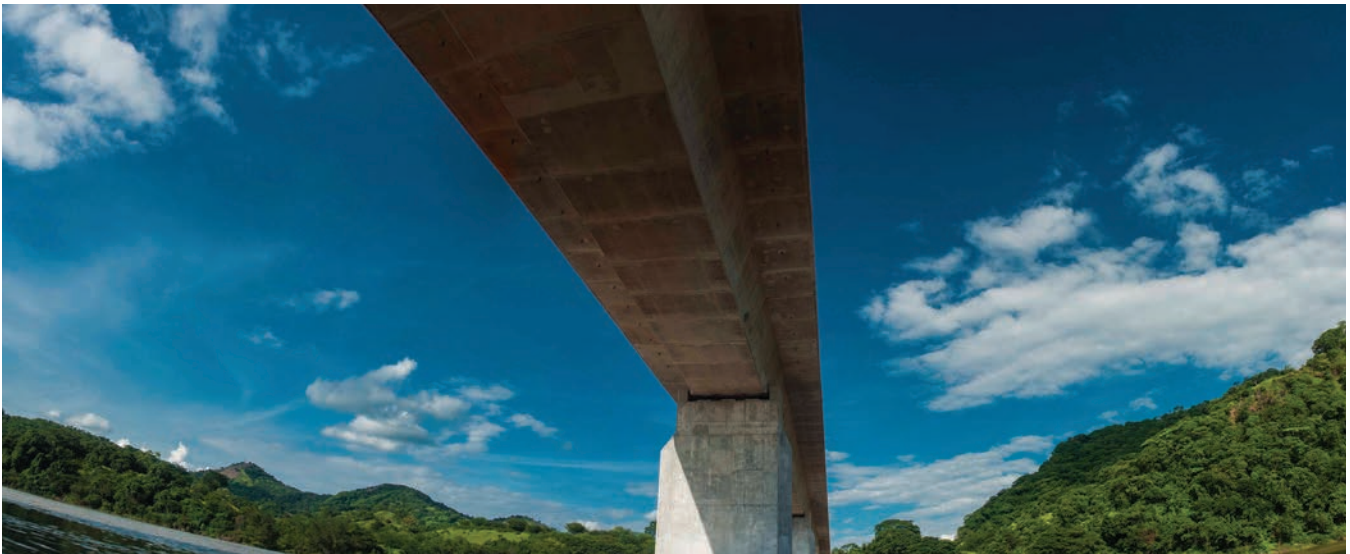
MCC's El Salvador Compact helped build several bridges to improve connectivity between the northern zone across the Sierra Madre mountains and the rest of the country. Credit: MCC
