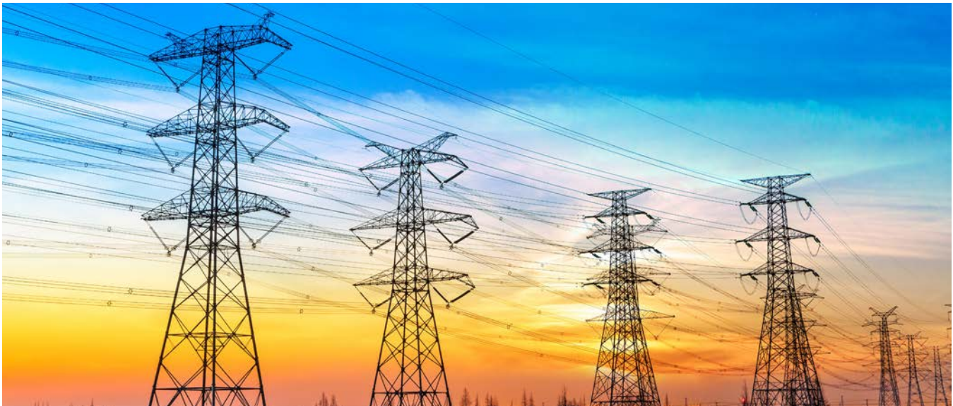
Electric transmission lines face risks from extreme heat and other climate hazards. Credit: Shutterstock
