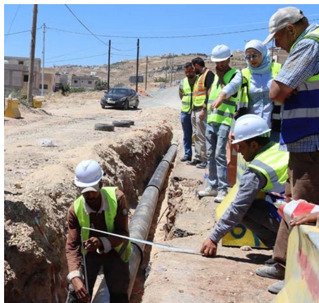
USAID Jordan improved the country's water supply network by replacing outdated components and installing smart meters and leak detection equipment. Credit: USAID
