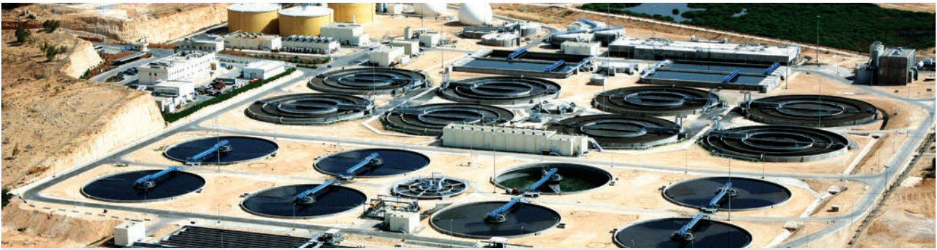
Through a public-private partnership, MCC assisted in the expansion of the As-Samra wastewater treatment plant in Jordan to increase its capacity and to provide freshwater to the water-constrained country's population. Credit: MCC
