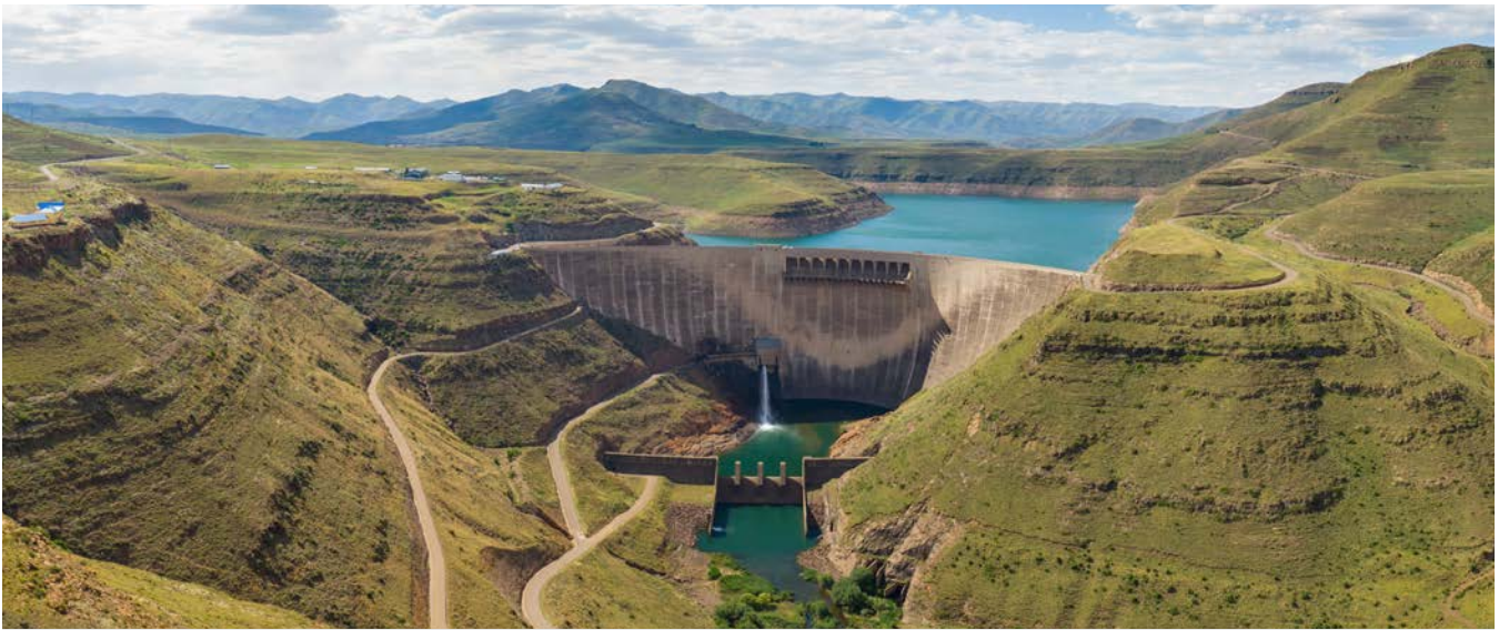
Dams exemplify how natural systems like rivers interact with built infrastructure systems such as energy generation. Credit: Shutterstock
