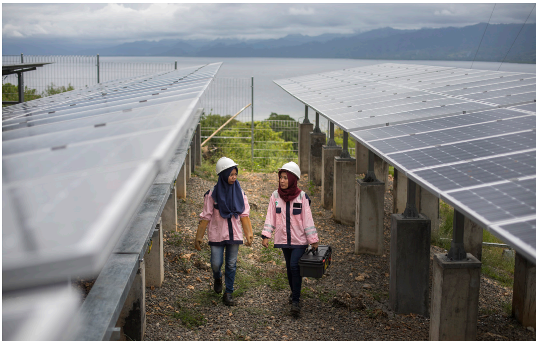
Junior electrical technicians inspect and maintain solar panels on Karampuang Island as part of the MCC-Indonesia partnership.
