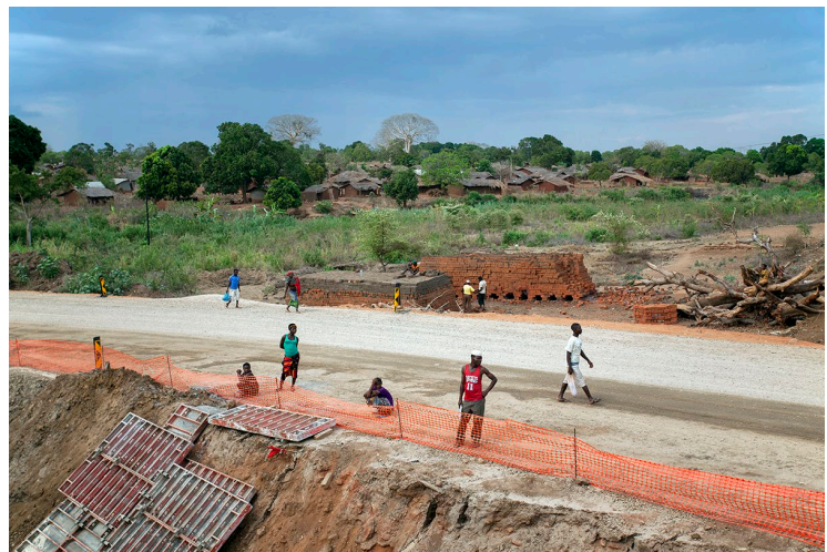
Road undergoing rehabilitation
