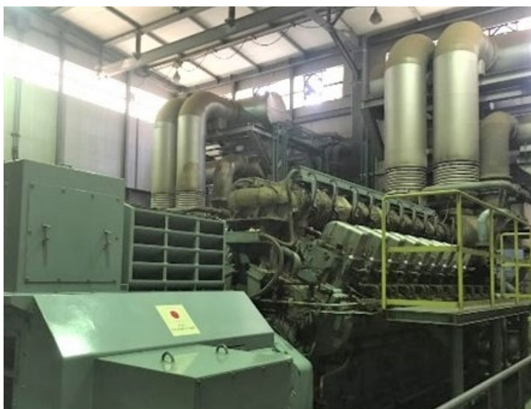
Kingtom thermal power station and the Generation Company's headquarters
