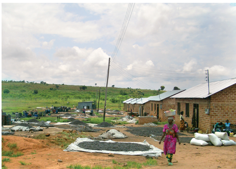
Power lines in rural Tanzanian community
