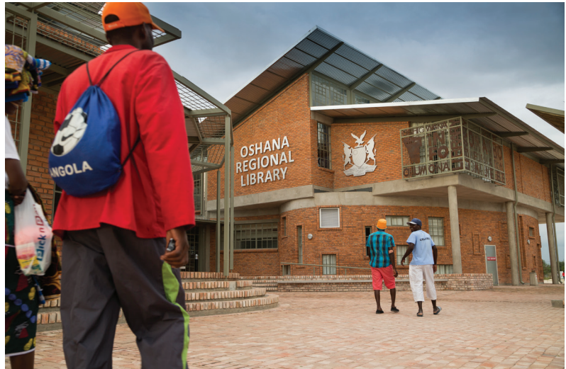
The Oshana Regional Library is an MCC-funded resource center in Oshakati, Namibia. Under the Namibia Compact's Education Project, MCC is constructing many regional resource and study centers like the one seen here in underserved areas in an effort to improve educational and professional outcomes.
