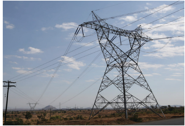
Transmission upgrades at the 400-kv Nkhoma Substation, completed as part of MCC's $350.7 million compact with Malawi
