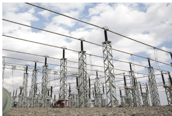
Construction nears completion at the 400-kv Nkhoma Substation, a significant transmission upgrade completed as part of MCC's $350.7 million compact with Malawi.
