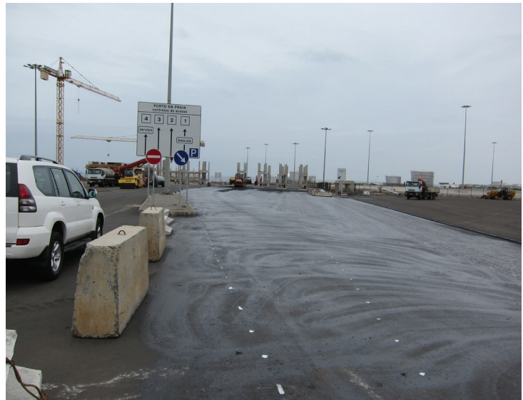
Construction and modernization of port entrance checkpoint.
