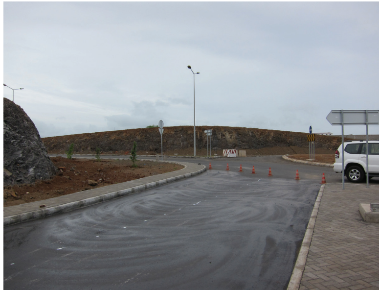
Port of Praia entrance - inbound & outbound road renovation & extension.
