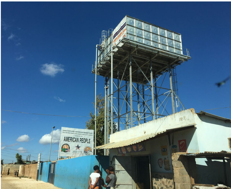
Newly constructed water tank
