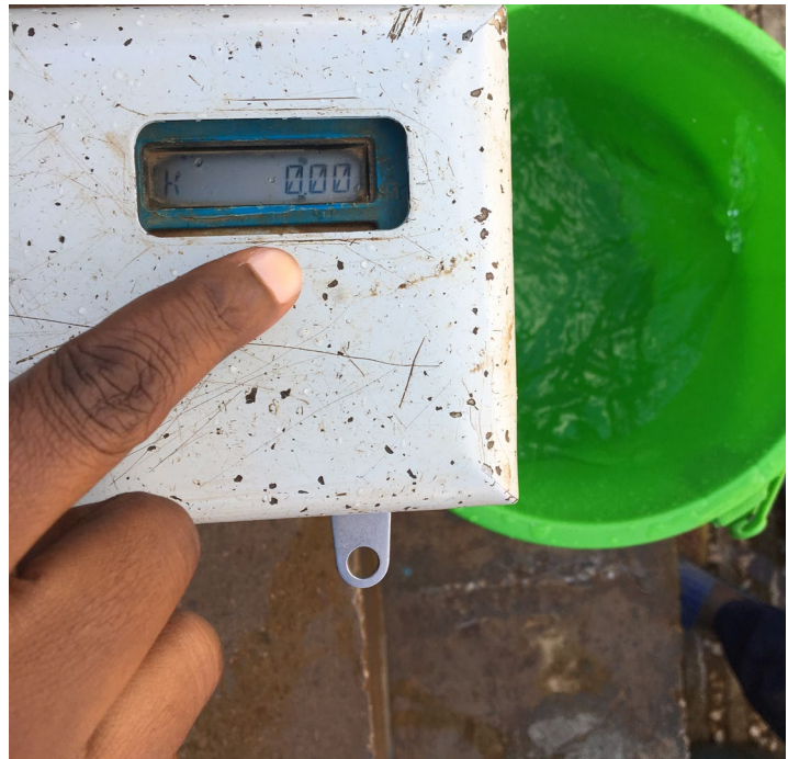
The newly installed kiosk token system in use
