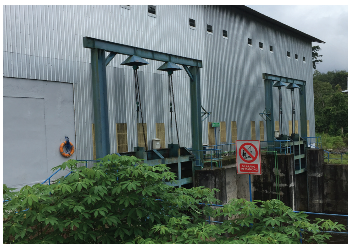
This power house was funded by one of the grants and is located near Sangar, West Padang Province.
