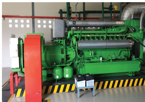
The palm oil biogas engine is one of the engines purchased through a grant. This one is location in Rokan Hilir district of Riau Province. Bahana Nusa Interindo Palm Oil plant.
