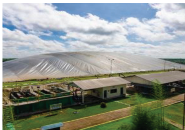
A palm oil methane effluent capture power plant funded by a Green Prosperity Project grant in Riau Province.
