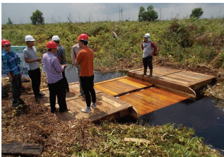
A wooden drainage canal blocking system in Berbak National Park, one of the two major designs to slow water movement in peatland drainage canals in an effort to rewet and restore peatland.
