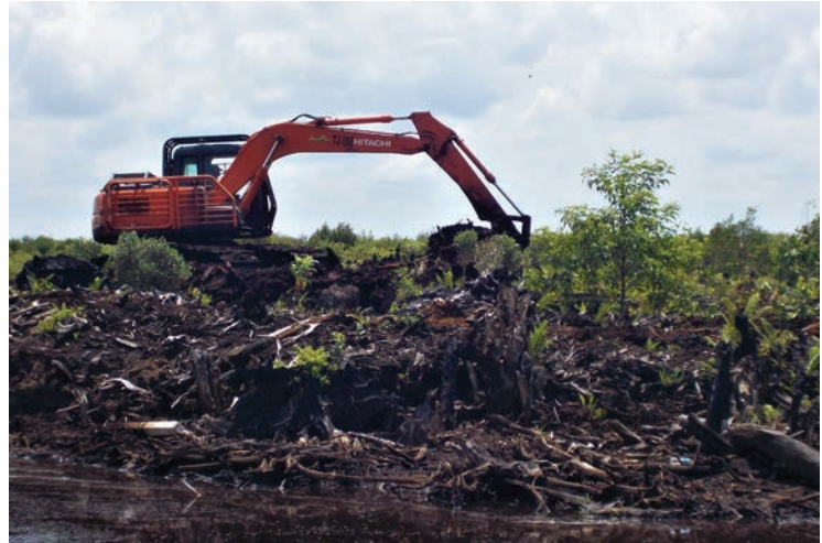
The second main method of blocking peatland drainage canals is to use dams made of compressed peat. Here a back-hoe moves peat into place to block a drainage canal.
