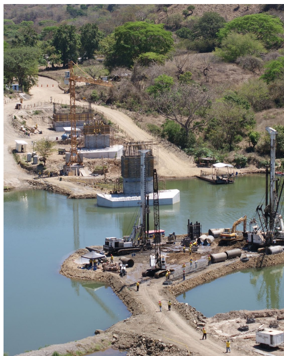
Constructing a bridge over the Lempa River
