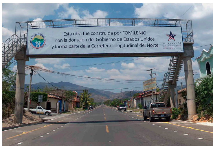
An improved section of the Northern Transnational Highway
