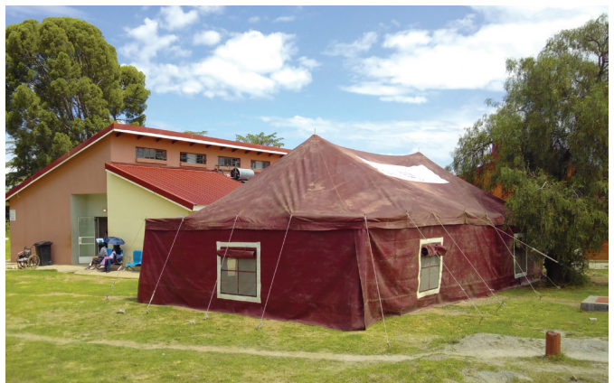
Tent Erected at MCC-Funded Outpatient Department in Mafeteng
