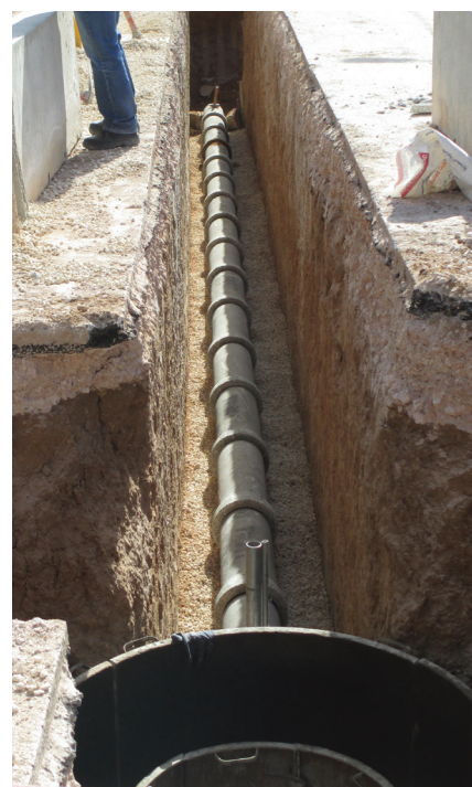
Construction of water network piping
