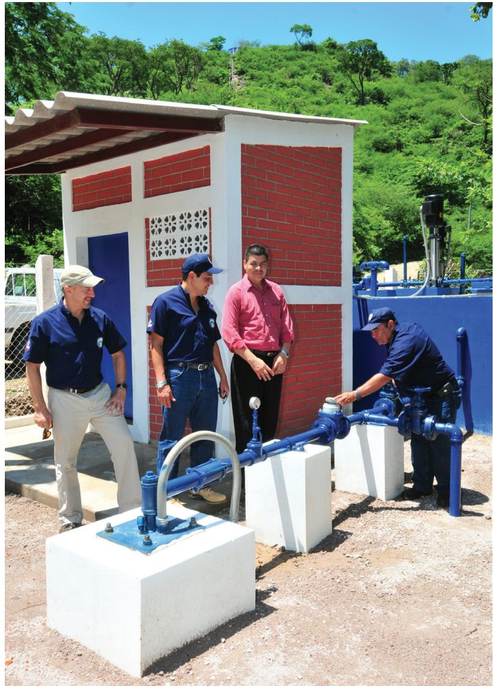
MCC and local implementing staff inspecting a new MCC water project.
