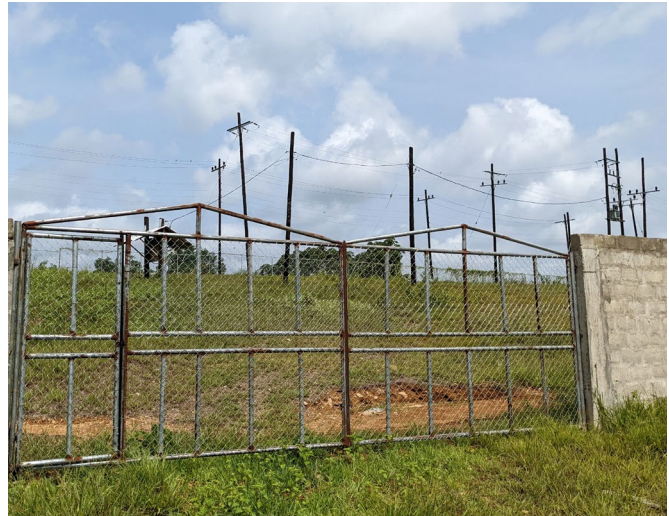
Outdoor Training Center at LEC with electricity poles used for training.
